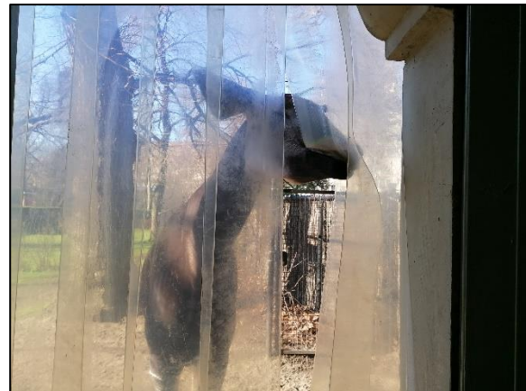
Figure 48 – Plastic strips on the doors are a good option to keep the indoor facilities insulated from cold weather while still allowing the animals to enter and exit the facility. ©Antwerp Zoo / Location: Antwerp Zoo
