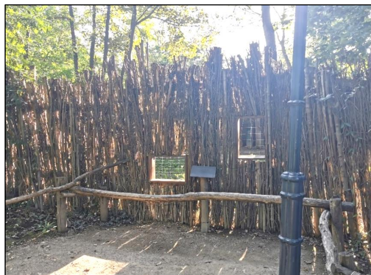
Figure 40 – Secondary barrier composed of small windows allowing the visitors to peek the enclosure while safeguarding the privacy to the animals. ©João Pedro Meireles / Location: Zoo Leipzig
