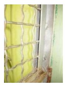
Figure: 14. Wave mesh welded between steel profiles (Photo: G. Fernández Hoyo)
