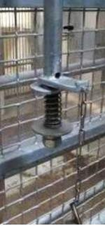
Figures 21 & 22. Sliding door that moves along a strip with teeth, fixed to the fence construction.
