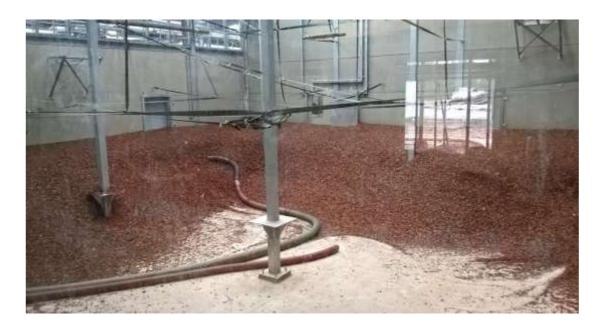
Figure: 25. Installing the bio-floor at Twycross Zoo (Photo Twycross Zoo)
