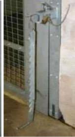
Figures 19 & 20. Sliding door with teeth on the handle as applied for orangutans at Chester Zoo.
